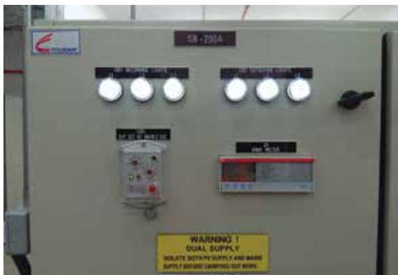
FIGURE 8.8 LED indicating grid supply and FPV supply
