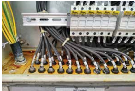
FIGURE 9.19 Water ingress and IP integrity compromised
