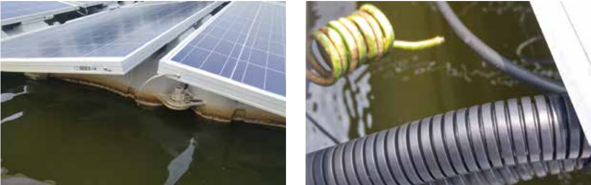
FIGURE 9.20 Bonding tapes/wires snapped due to constant motion of floats and excessive slackness
