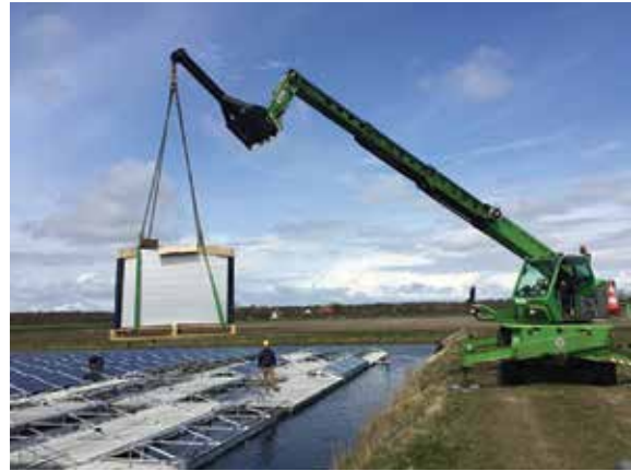
FIGURE 7.3 Two ways to assemble and launch floating PV structures: on a ramp or in the water
