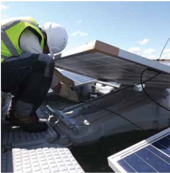
FIGURE 9.14 Corrective maintenance carried out on the float
