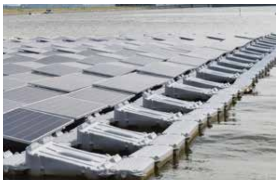
FIGURE 9.23 Varying tilt angle induced due to wind and waves
