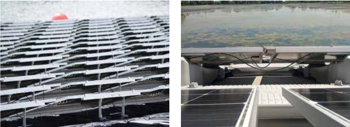
FIGURE 9.21 Grounding cable run—series layout (left) and parallel layout (right)
