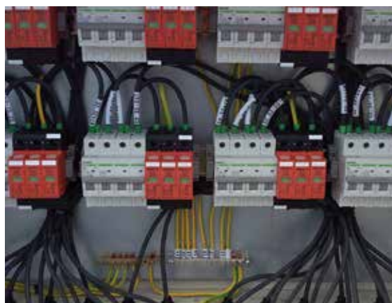
FIGURE 8.2 DC cabinet with surge protection devices (red-orange)
