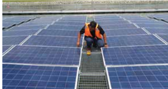
FIGURE 8.5 Solar professional performing continuity tests
