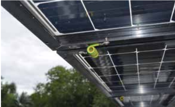
FIGURE 4.17 Equipotential bonding, Singapore Tengah Reservoir testbed
