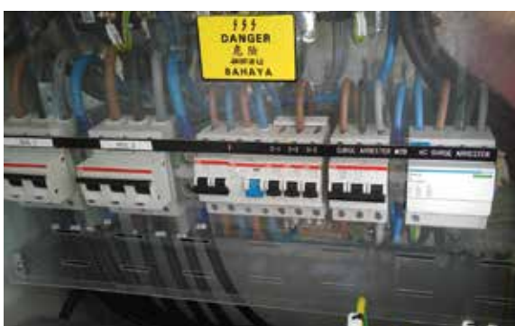
FIGURE 8.9 AC subboard with surge protection device
