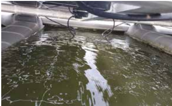
FIGURE 9.15 Connectors and cables submerged in water
