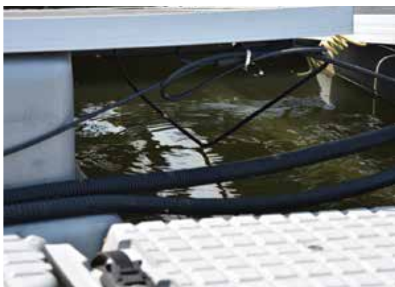
FIGURE 7.6 Examples of cables in contact with water
