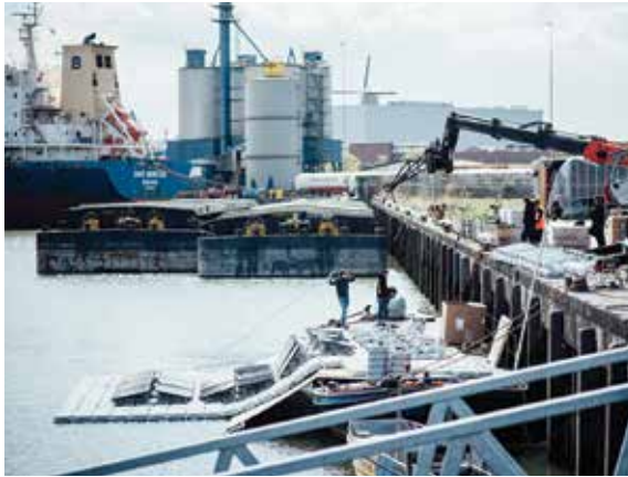
FIGURE 7.3 Two ways to assemble and launch floating PV structures: on a ramp or in the water
