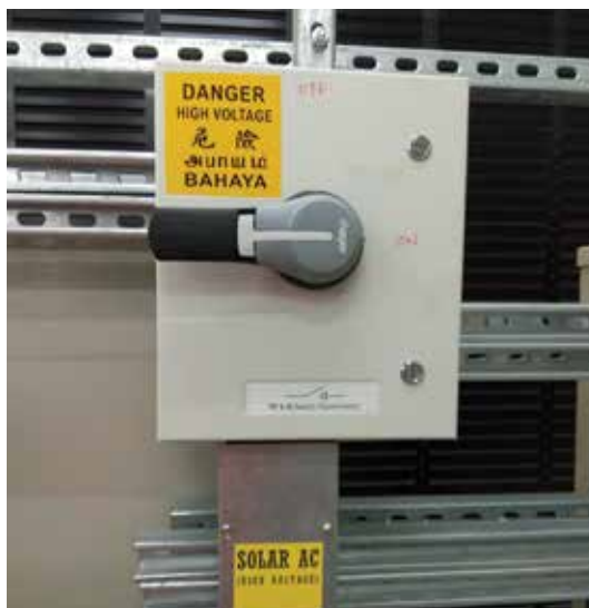
FIGURE 8.10 AC isolator
