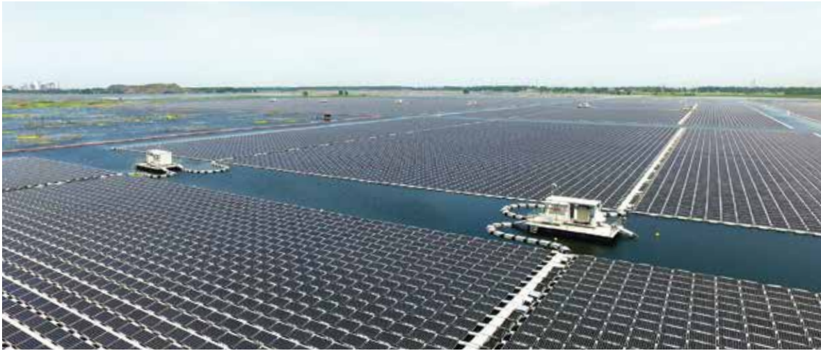
FIGURE 4.1 Central-inverter configuration for FPV systems, China
