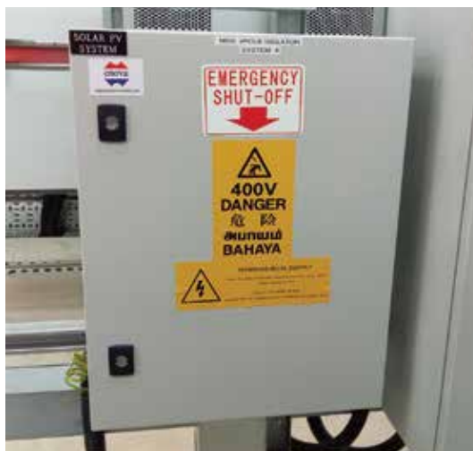
FIGURE 8.11 AC isolator with emergency shutoff
