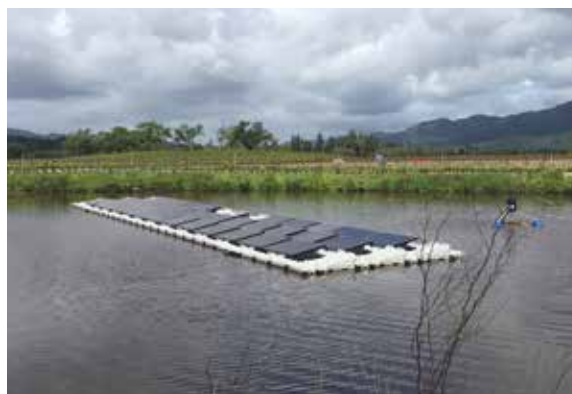
FIGURE 1.2 Examples of floating photovoltaic systems: 150MWp in Guqiao, China (left) and 10 kWp system in Kunde winery, California, United States (right)
