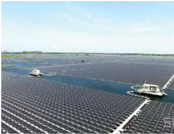
FIGURE 2.13. Sungrow FPV farm with a central inverter on a floating island (left), detailed view of the floating island for the central inverter (right)
