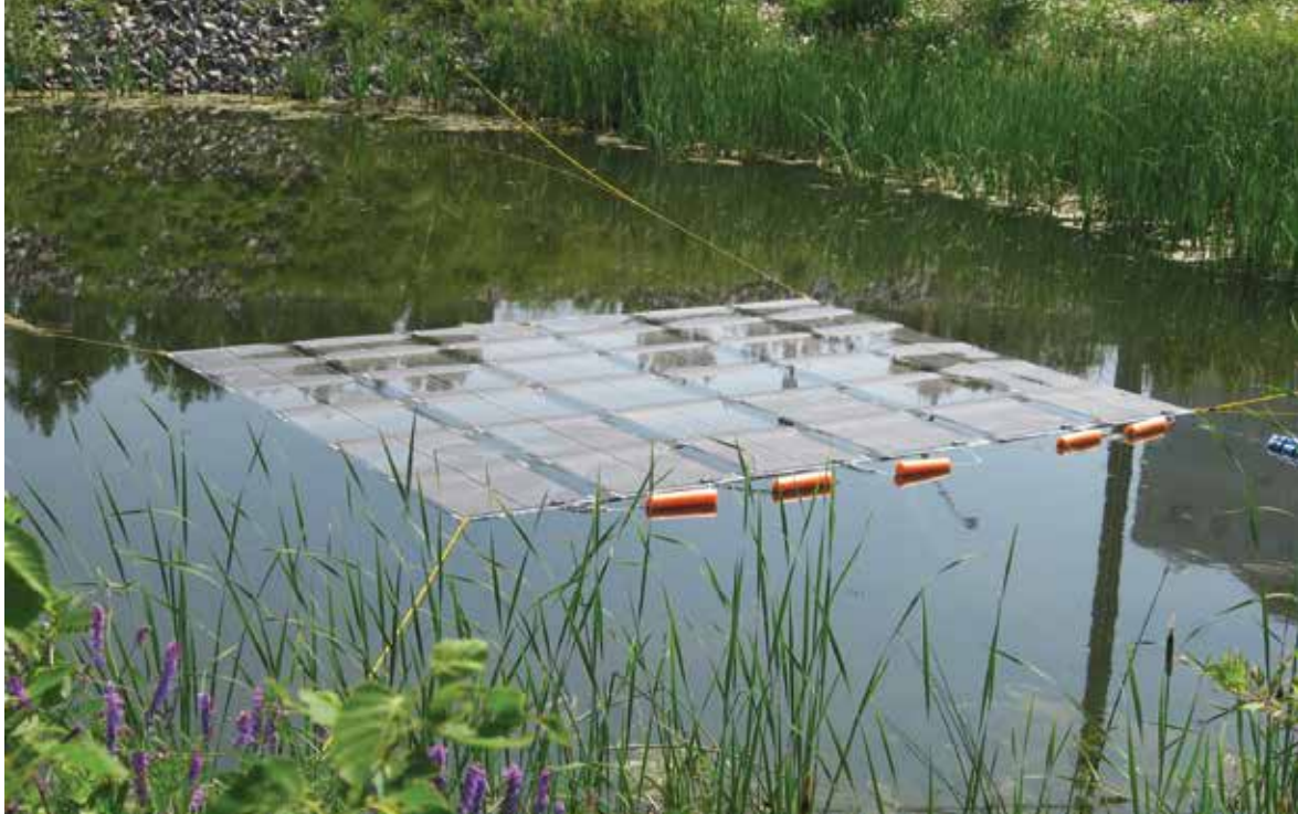
FIGURE 2.21. The 0.57 kWp MIRARCO Mining Innovation semi-submerged floating thin-film system in Sudbury, Canada
