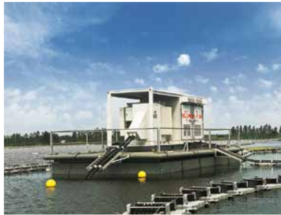
FIGURE 2.13. Sungrow FPV farm with a central inverter on a floating island (left), detailed view of the floating island for the central inverter (right)
