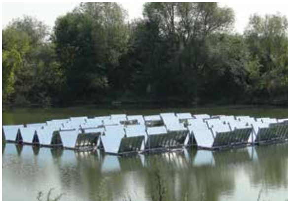
FIGURE 2.17. Low concentration with V-shaped mirrors for FPV
