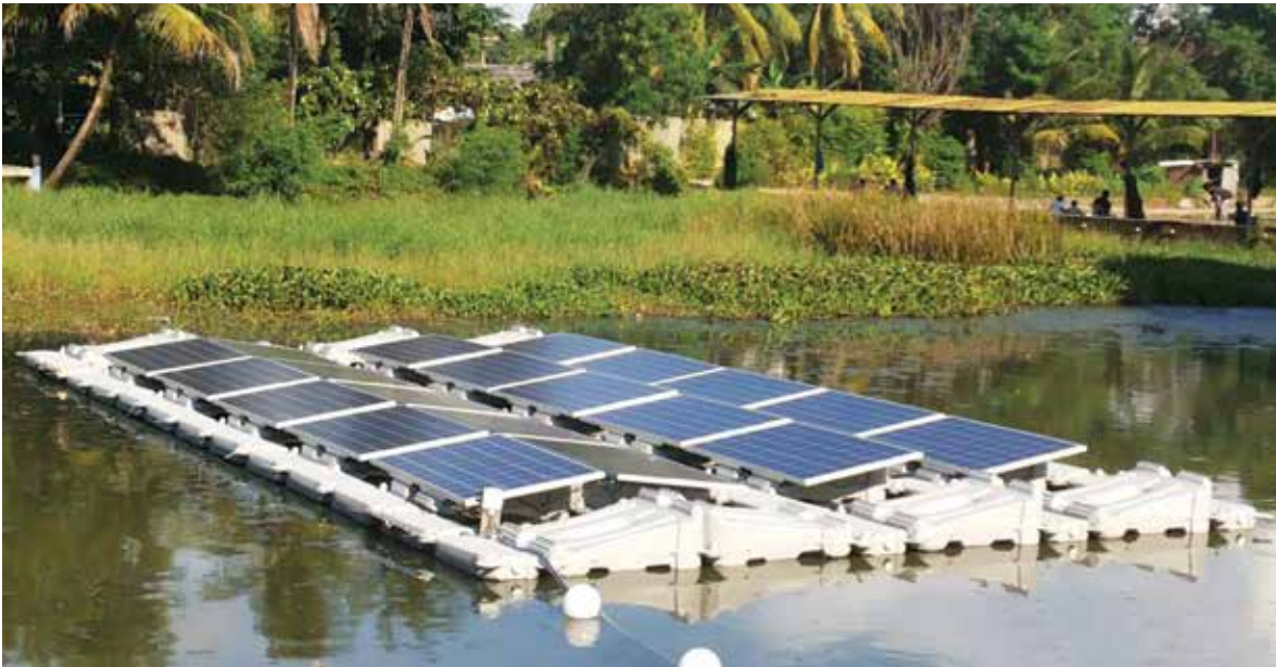
FIGURE E.2 The most common float types: pure float, Indonesia (top) and pontoons with metal structures, India (bottom)
