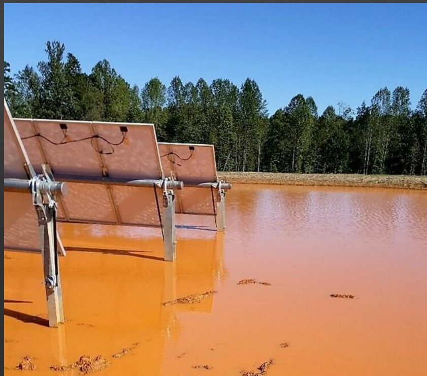
Actual site with NX Horizon post-Hurricane Matthew. Slew gear, motor and electrical components untouched.
