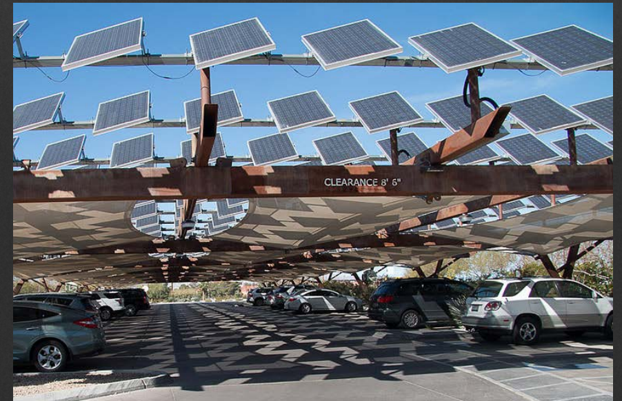
PowerLight tilted 1 axis tracker over reflective fabric with Sanyo HIT. Springs Preserve 2008
