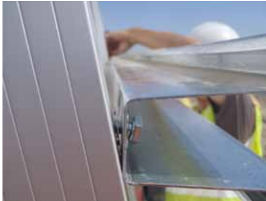
Shown loose and with optional WEEB-UIR – torque as per construction documents
