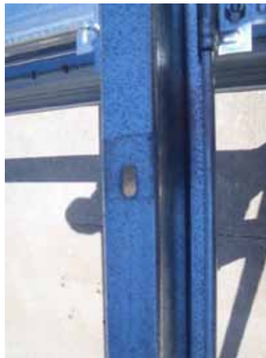
Slotted hole in NS Beam used for connection to modules
